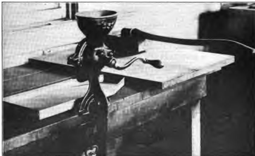
Figure 2.—COAL GRINDER OF THE COFFEE-MILL TYPE.
